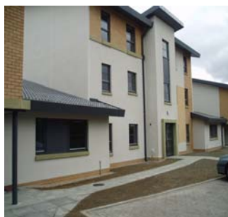
North Shore lane, Troon - 4 Houses and 20 flats
