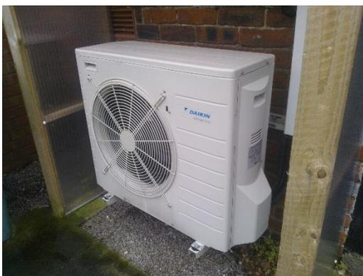
Fig. 7 Outdoor component of ASHP as installed at the Hadyard Terrace properties
