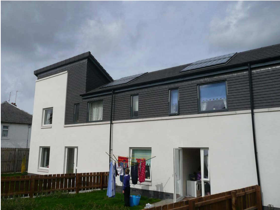
Plate 2 South elevation of units 7b and 7c
