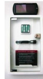
Situated on the communal landings, these boxes contain torches for viewing inside the poles, and are recharged by a solar panel.
