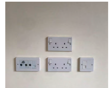
Double socket, USB outlet, TV/satellite and BT point within Living Room/Bedroom 1
